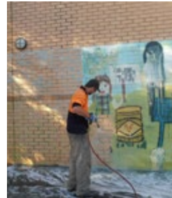
Mural removal after spraying TRANSGEL with airless paint sprayer.
