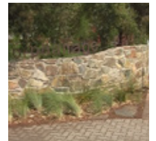
Once clean, re-apply WBGC.
